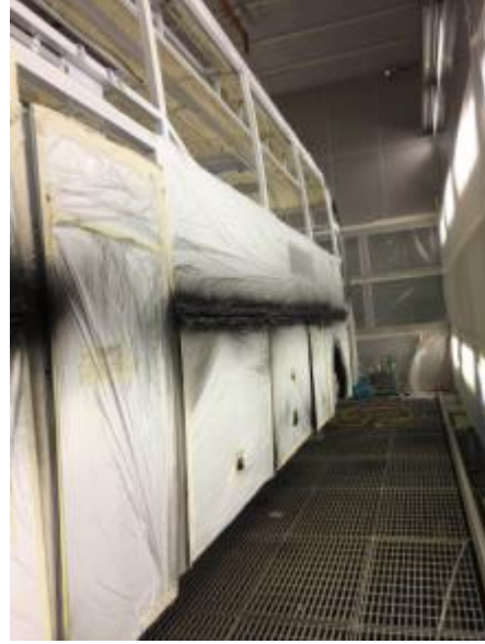
Fig. Painting the inner surface of the skin
