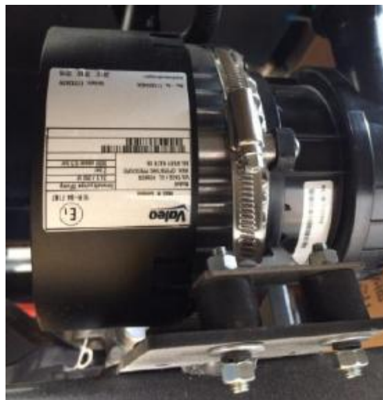
Fig. Installation and fixing position of water pump
